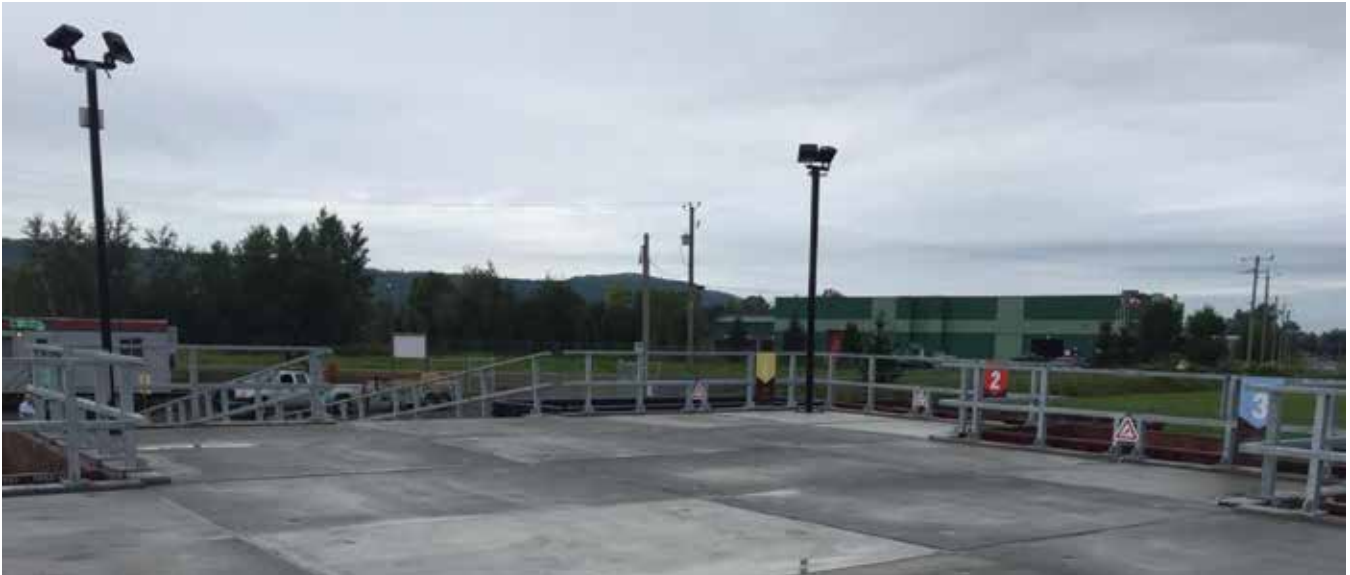
Modular residential drop off solution for Rigaud, Quebec.
