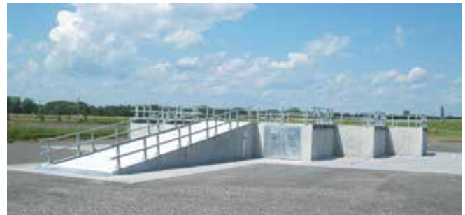
Modular residential drop off solution for Rigaud, Quebec.
